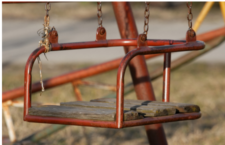
Open “S” Hooks and Defective Seat.
