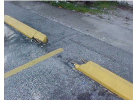
Insure there is no protruding rebar.
