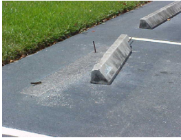
Insure parking stops are properly secured in place.
