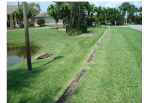
Ensure all parking stops are sufficient height to prevent cars from driving into the lake.
