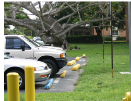
Note disabled parking stop and others not secured.
